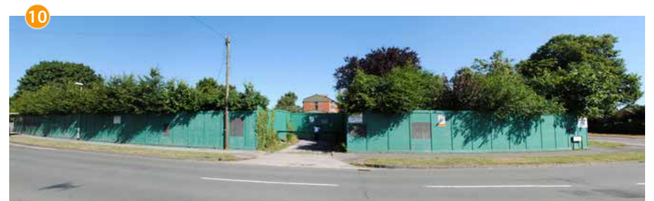
Looking towards the site corner at the Dwyer Road/Burghfield Road
